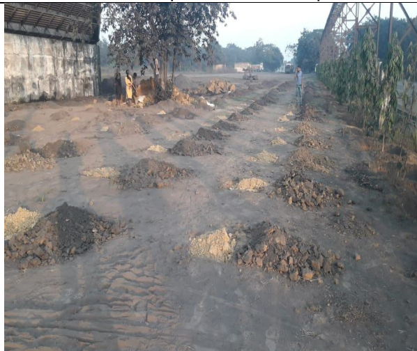
Plantation is being done near cooling tower
