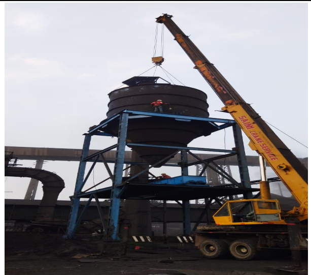
Ash silo dust collection installation work
