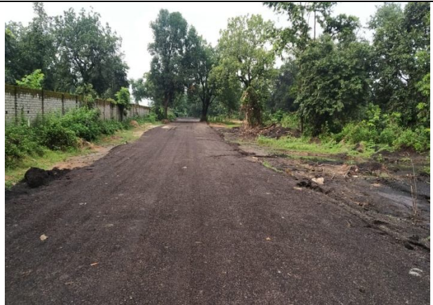
Road construction with SMS Slag near plant
