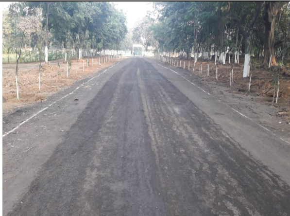
Road construction with SMS Slag in the plant
