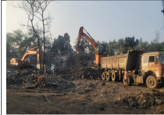
SMS Slag stock area cleaning work
